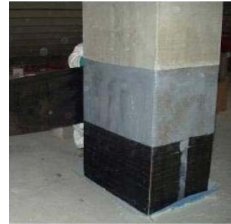
Fig 1: FRP for retrofitting of RC columns [8][13][11]
