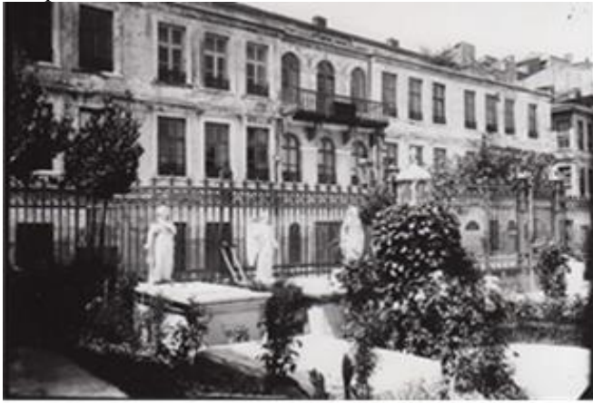
Figure 3: The structure of the Convent ended in 1850. Point of view from the churches' court. CSA, F. 1459 K, Inventory 1, Archival Unit 99.
