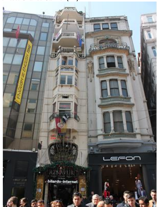
Figure 7: The façade of Aznavur passage in Istanbul.
