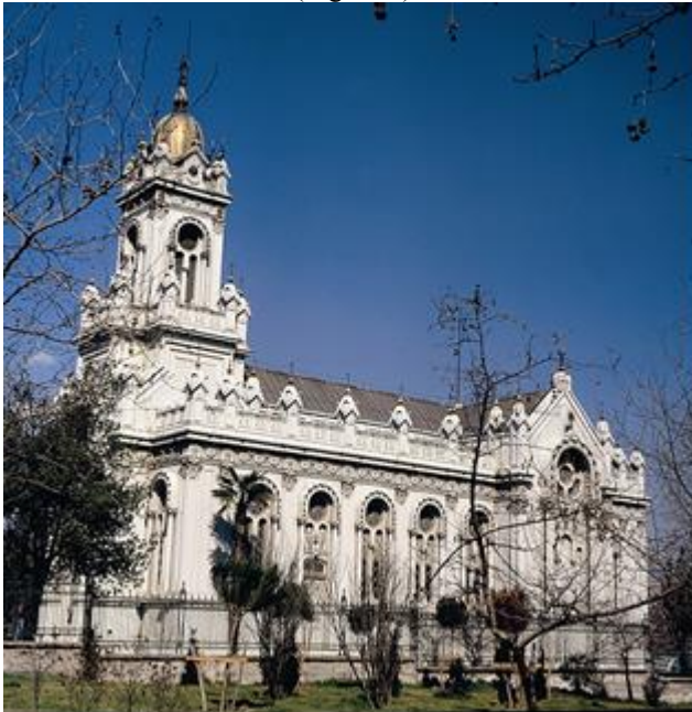
Figure 6: South façade of the St Stefan Church.
