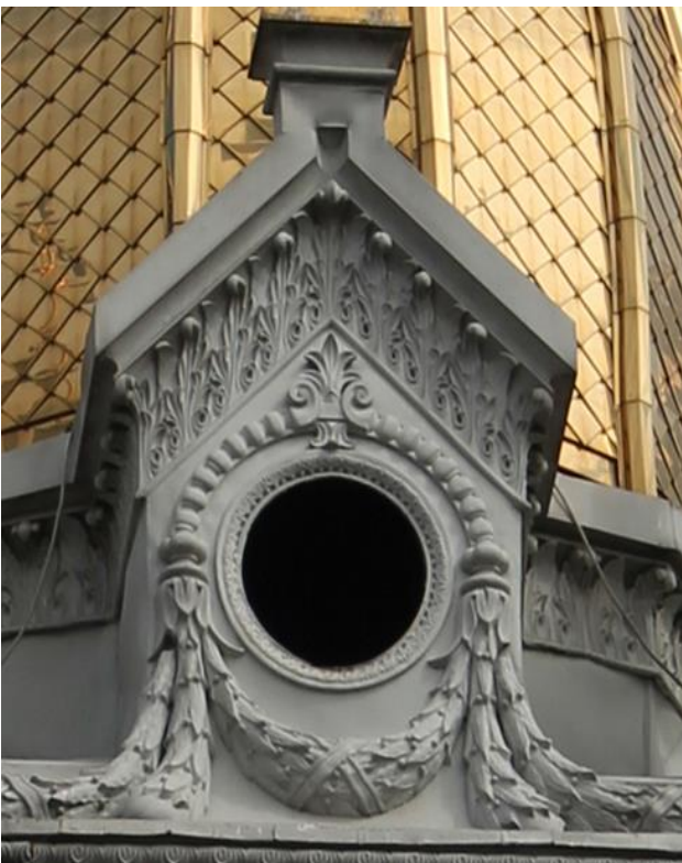
Figure 9: Cast-iron decoration of the dome
