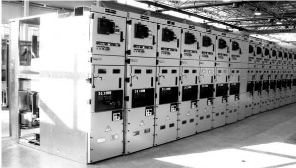
Fig. 2. 20 kV metal-clad switchgear (indoor switchgear equipment). [3].
