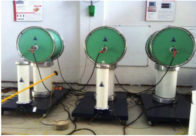
Fig. 2 Three Potential Dividers and Three Current Transformer
